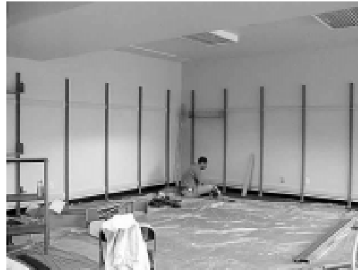
Library shelving going in by Guy
