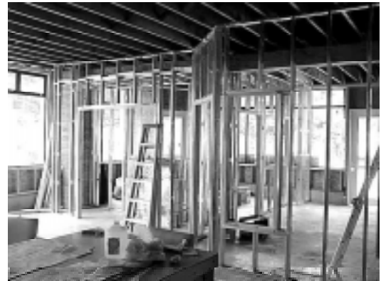
Framing in multipurpose room looking north
