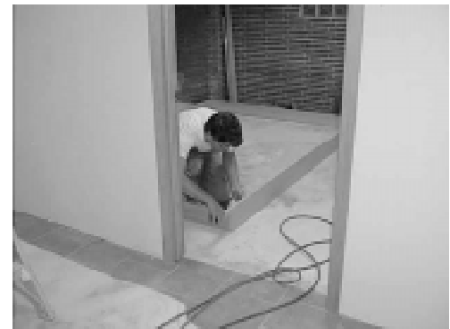
Window trim in progress by David
