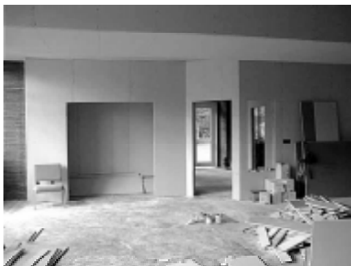
Sheetrock in multipurpose room
