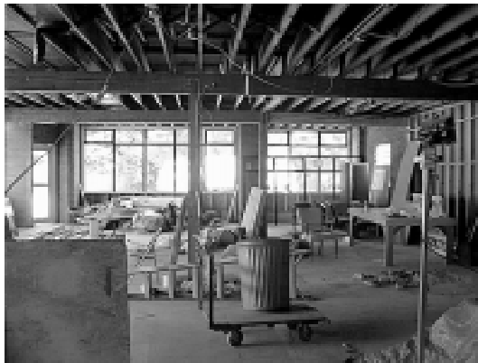
Empty shell looking north
