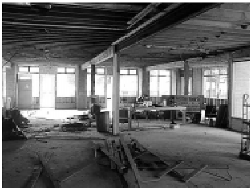
Empty shell looking west
