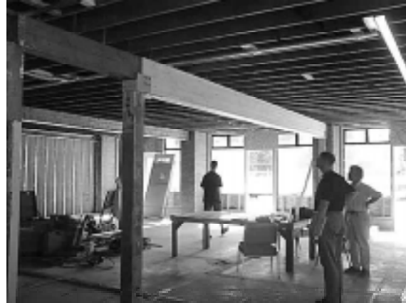
The multipurpose room big beam just installed
